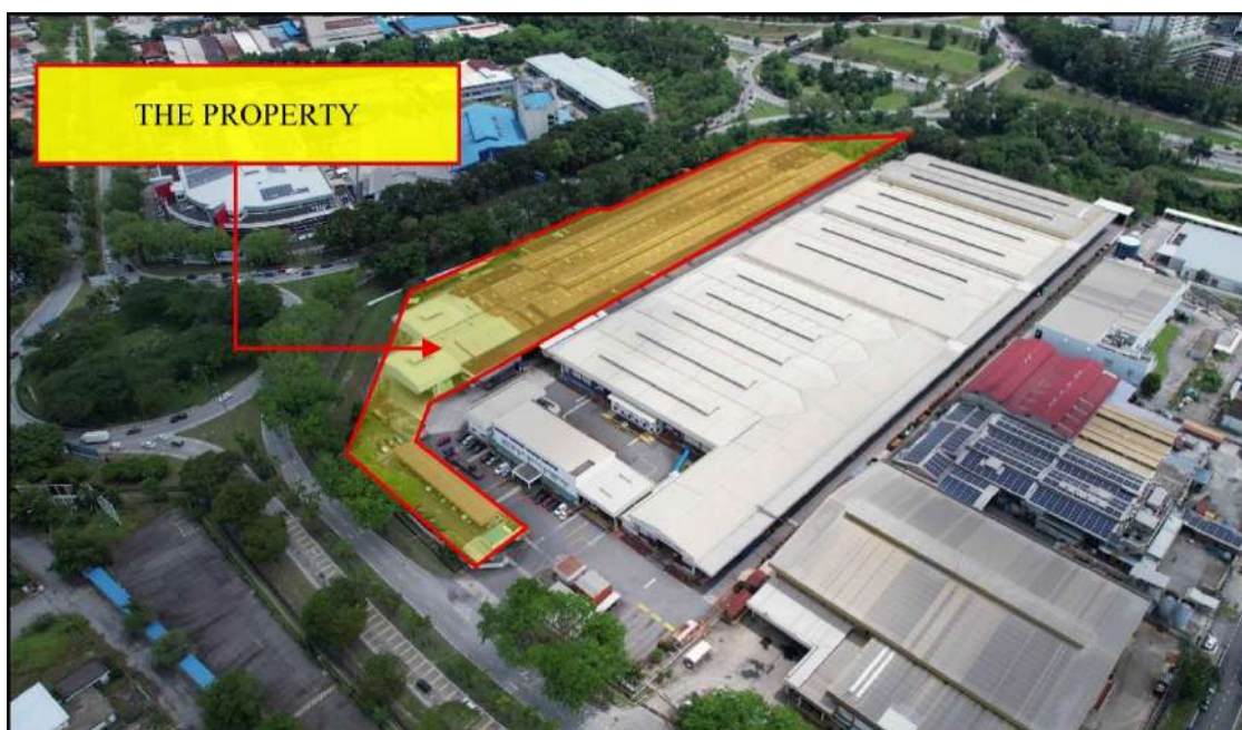
(Aerial view of the Property)
