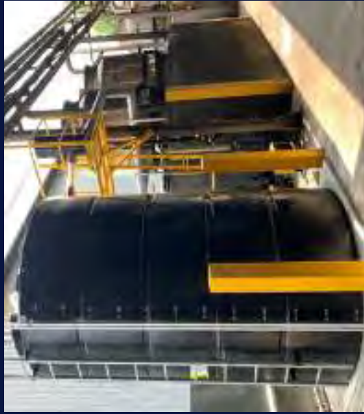
Installation of Rainwater Harvesting System
